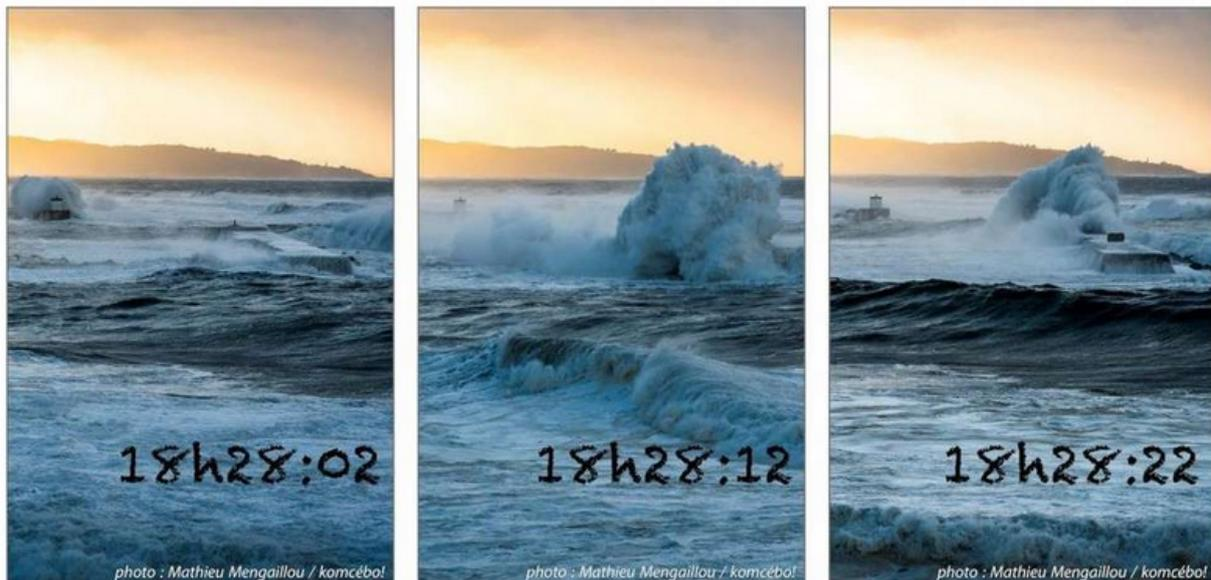
Figure 1: Photo of the ejection of a 50 T block on February 28, 2017
