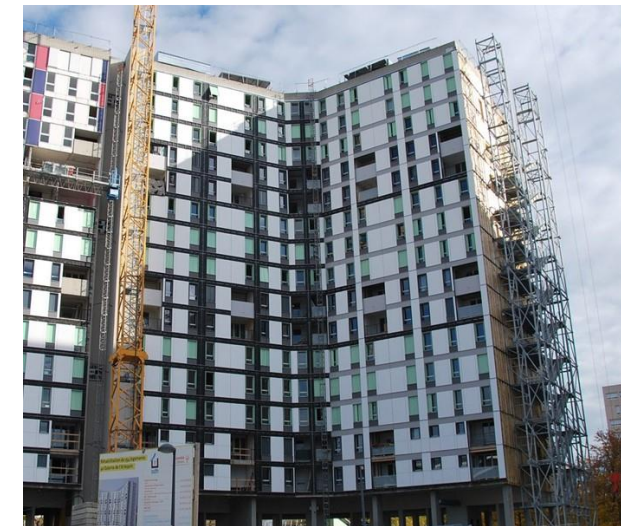
Rénovation R+15 in Grenoble by Techniwood
