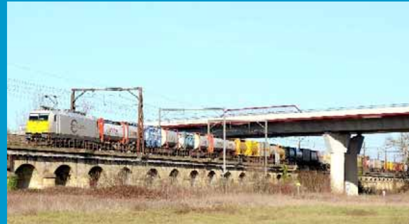
Viaduc des Cent Arches, Libourne (1848-1850) _ built on pine piles
