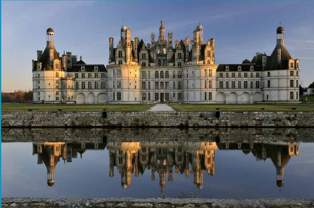
Château de Chambord built on oak piles (ar. 1520)
