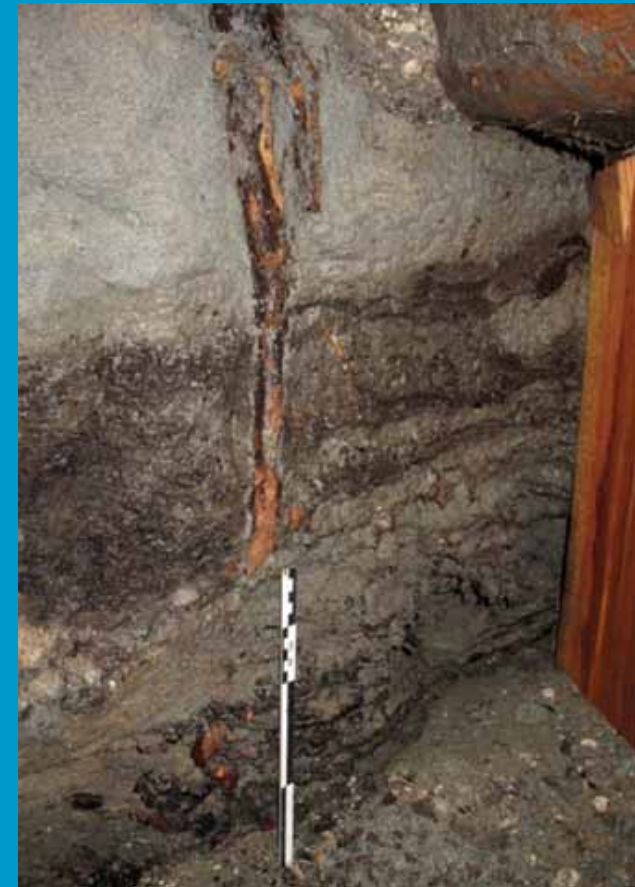
timber pile [BRYANT et al., 2007]
