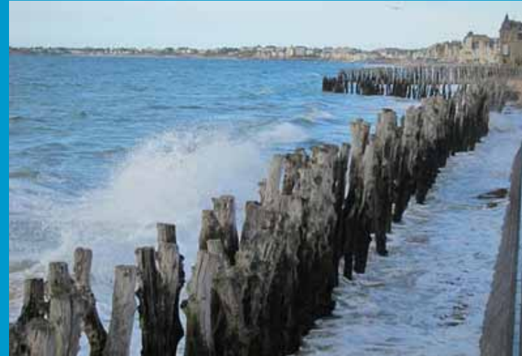
Oak timber breakwater, Saint-Malo
